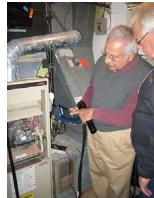
Inspecting HVAC equipment
